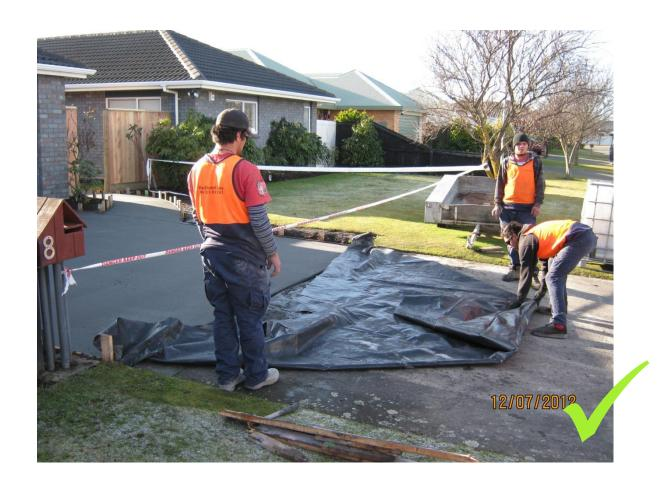
The polythene is then rolled out to create a bunded area at the bottom of the driveway.
