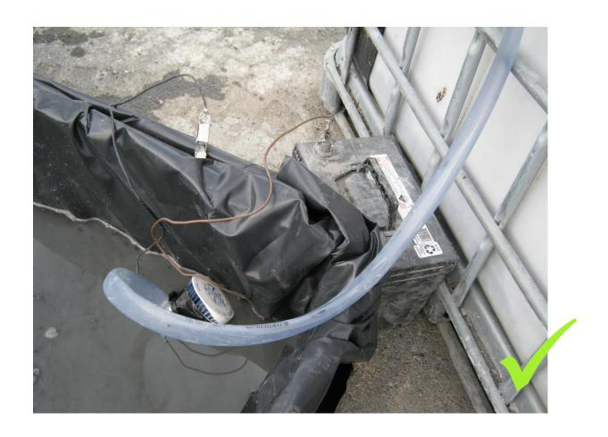
Contaminated wash water pumped into an IBC, sediment is kept in the bund.
